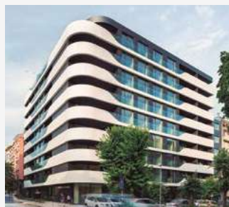
Varna Wave Building. Residential building. Varna, Bulgaria. Aquarea and Aquarea Smart Cloud.
