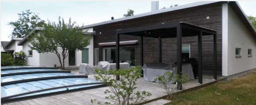
Single family house. Höllviken, Sweden. Aquarea with natural refrigerant R290.
