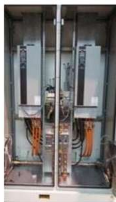
Compressor drives + main power connection
