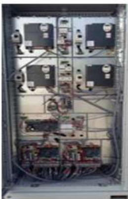
Fan drives + Pump drives + electronic boards
