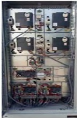
Fan drives + Pump drives + electronic boards
