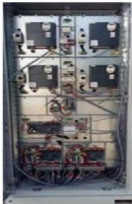
Fan drives + Pump drives + electronic boards
