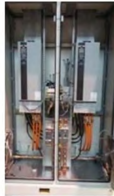
Compressor drives + main power connection
