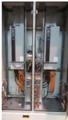
Compressor drives + main power connection
